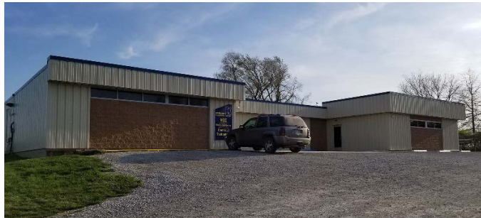
HCC - Electrical Building, 17349 Country Club Road, Atchison, Kansas
